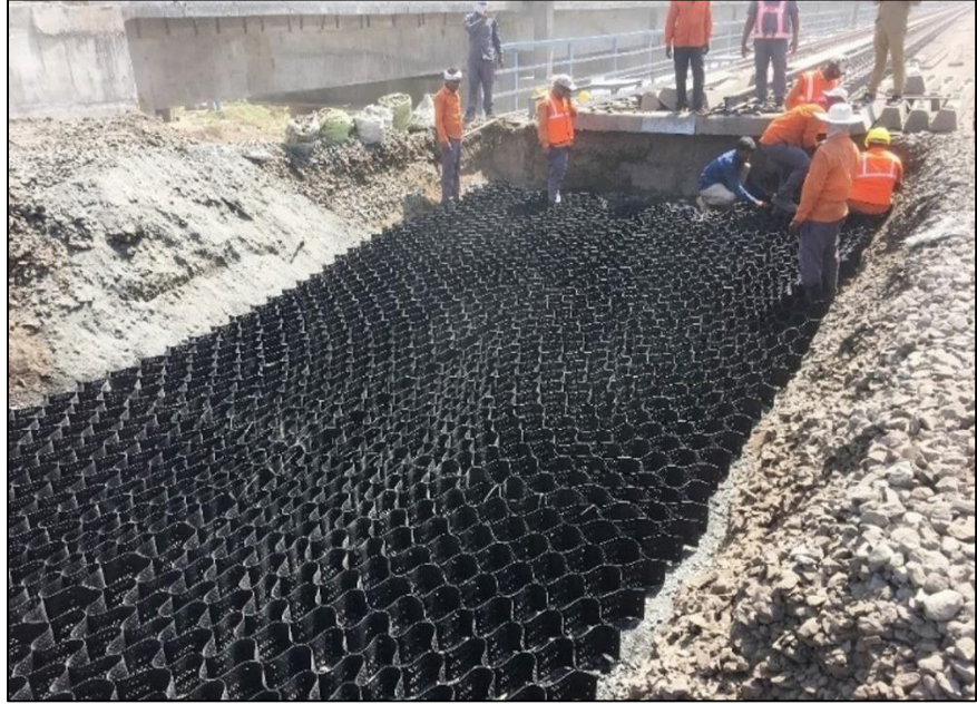
Geocell used as Approach slab in Western railways, Mumbai project
